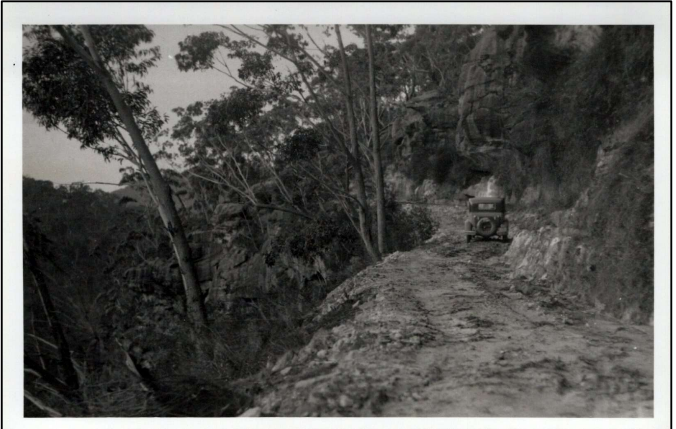
Part of original road off present Mt Irvine Road - known as "Arkensall" track (97/27)
