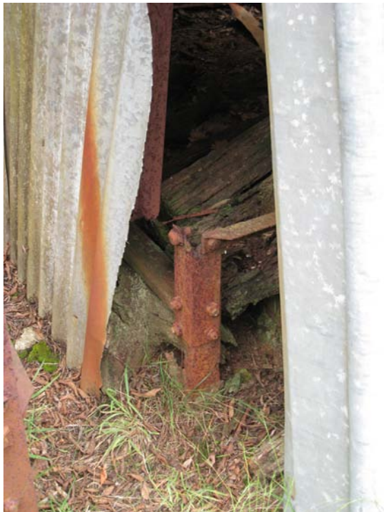
Figure 21: Severed leg at base of tank stand.
