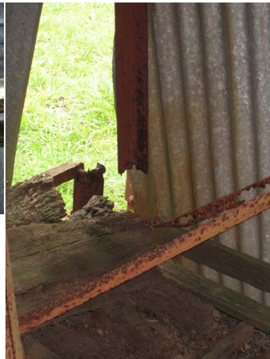
Figure 18: Severed leg at base of tank stand (of the eight tank stand legs, only three are providing support).
