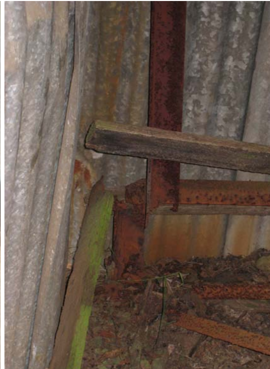
Figure 20: Severed leg at base of tank stand.
