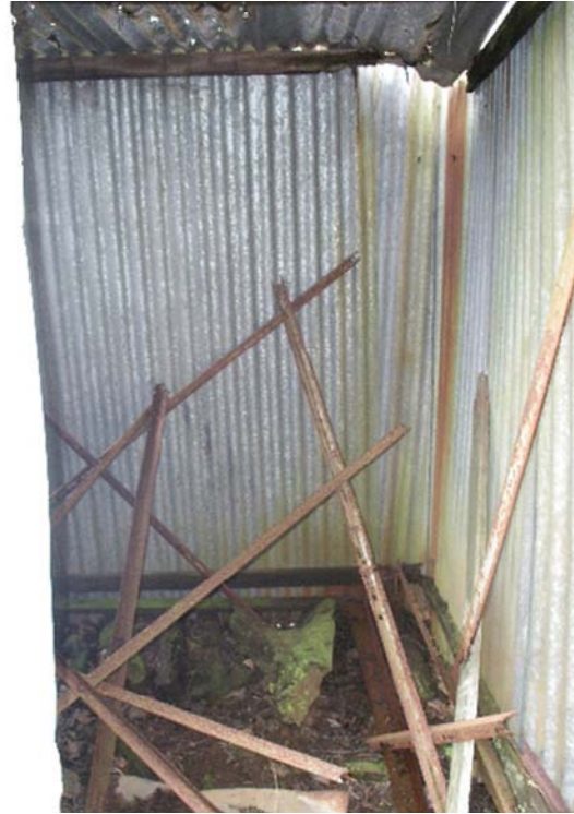
Figure 16: Corroded framing members. (Source: Hughes Trueman 2009)
